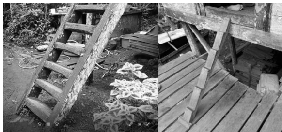
Fig 2. The stairs to the terrace (left) and into (right) the traditional house of Dayak Tomun
